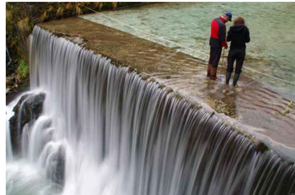
Flood control measurements of Fagli stream, Equi Terme (MS), Alpi Apuane, photo by M. Faverjon.
